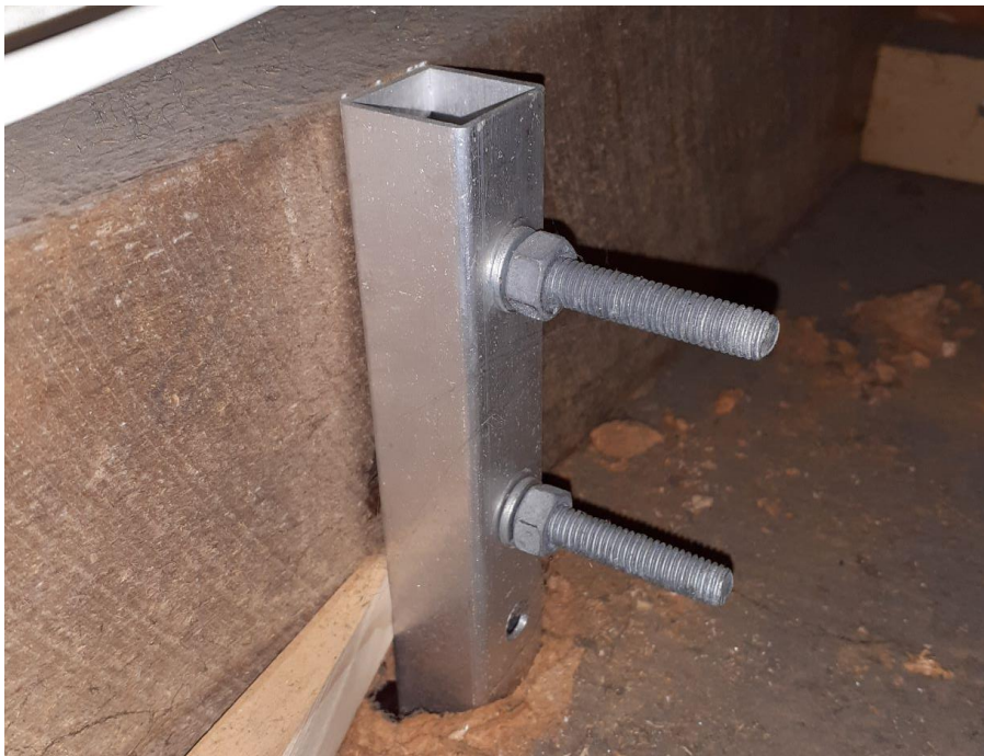
Photo of strut to rafter connection.
